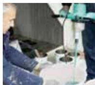
12. Miscelare Triflex Stone Design S e Triflex Stone Design R 1K.
